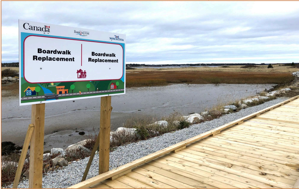
North East Point Boardwalk, District of Barrington, NS
