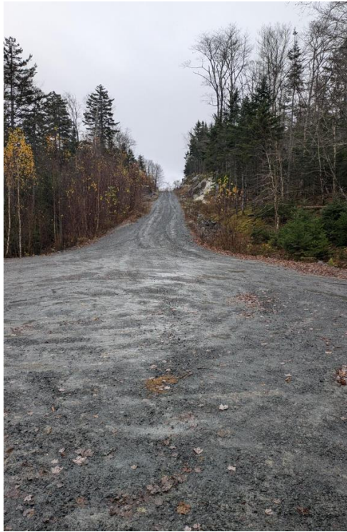
Long Lake Water Access Driveway
