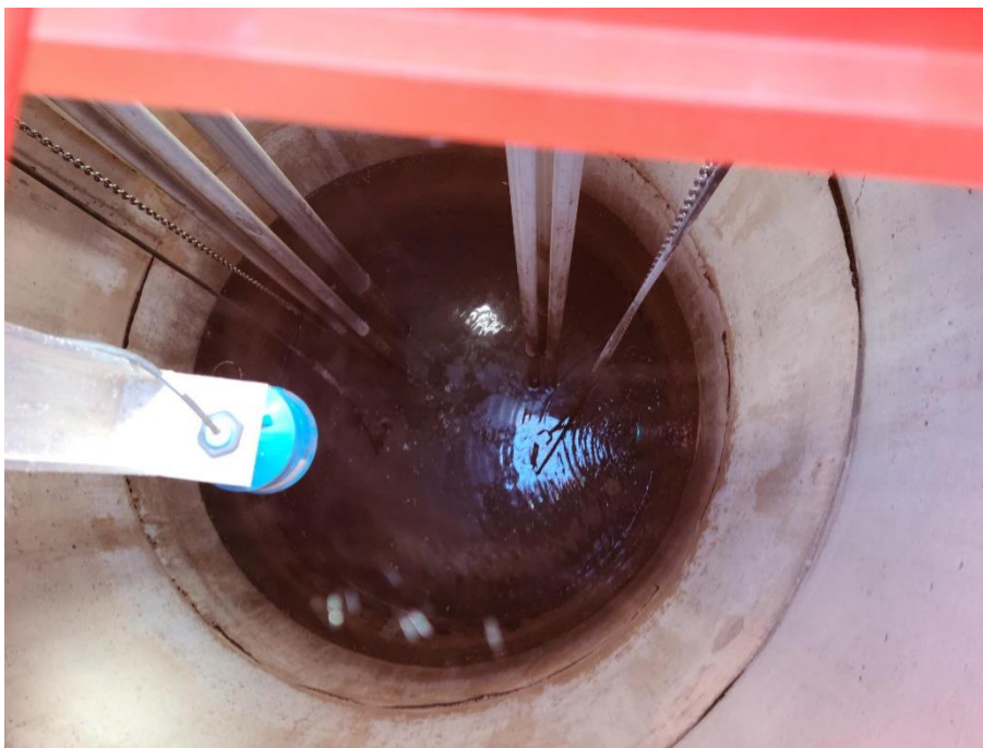
LS #11C: Park Road Extension - Inside of Wet-Well
