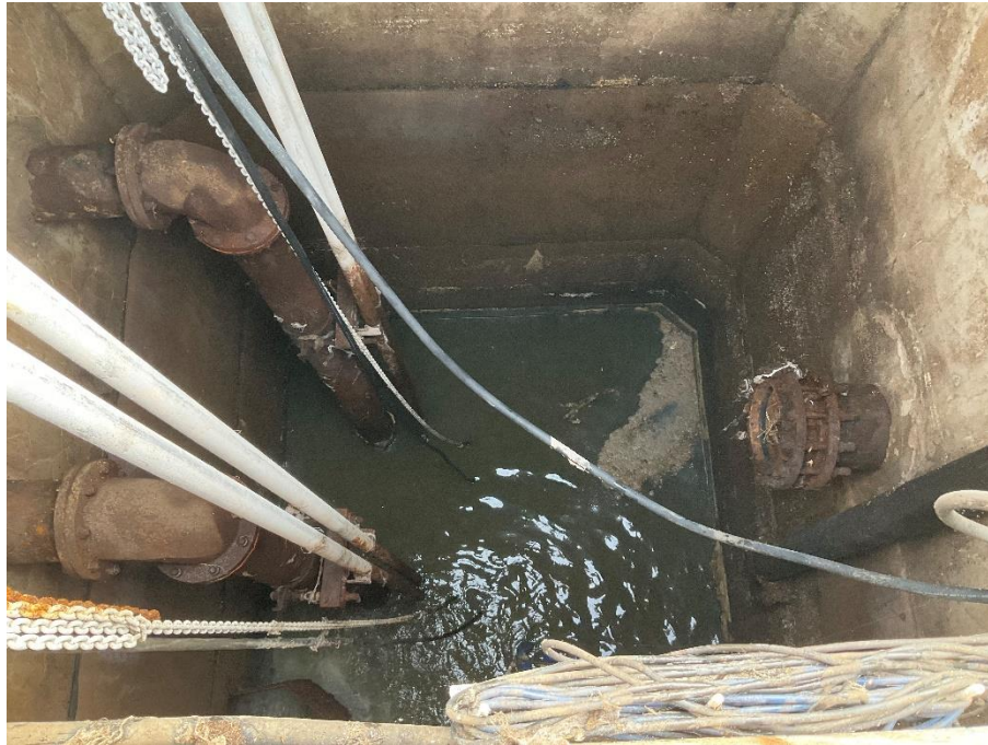
LS #17: Old Public Works Shed - Inside of Wet-Well
