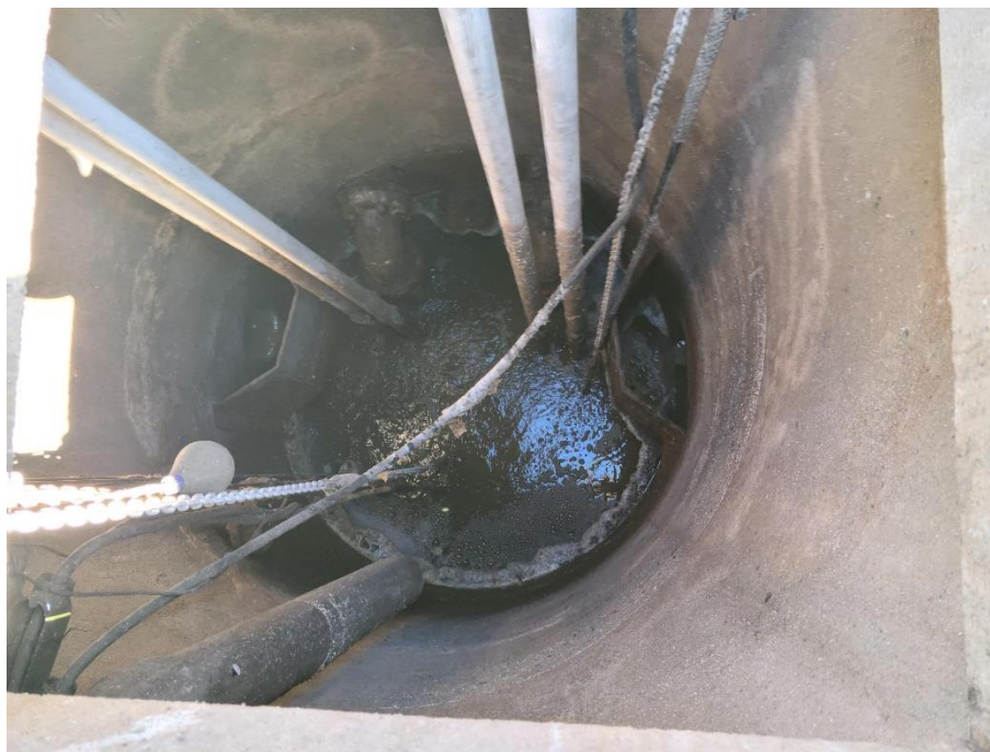
LS #10: Medical Centre - Inside of Wet-Well
