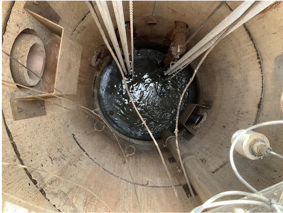
LS #23: Maitland Road - Inside of Wet-Well
