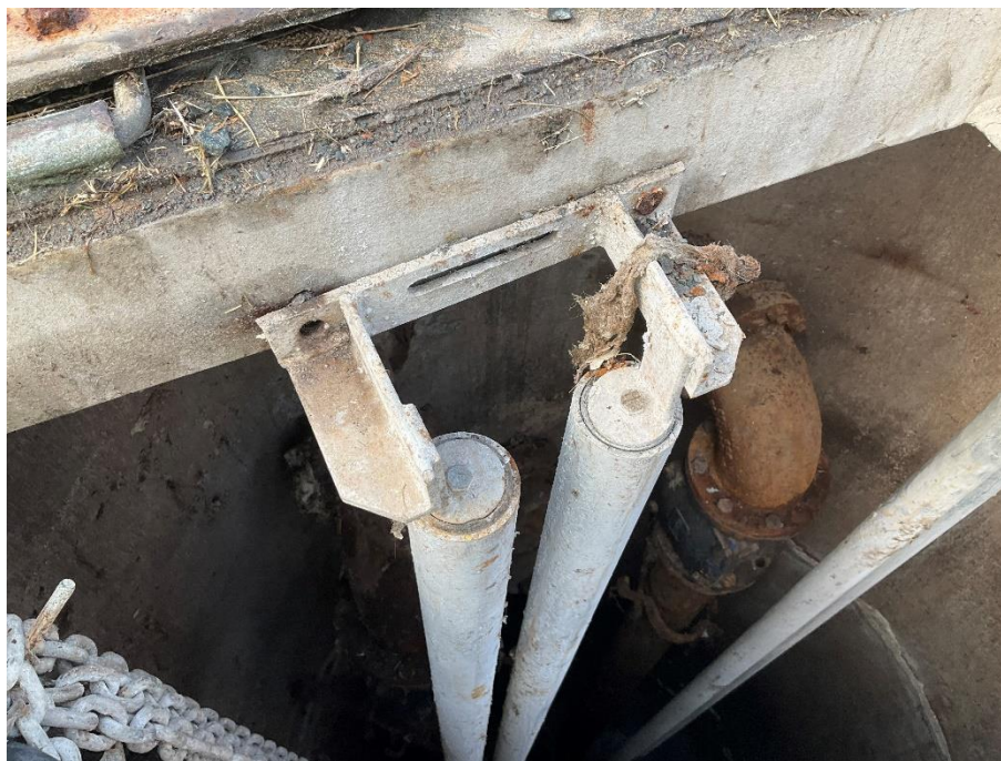
LS #18: Barney Brook - Loose guide rail bracket
