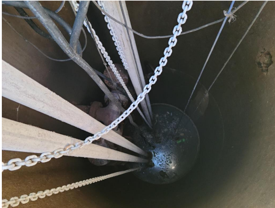
LS #10A: Pine Grove - Inside of Wet-Well
