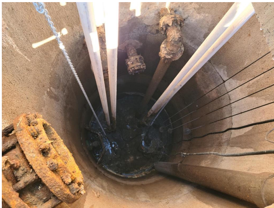
LS #12: Elmsdale Legion - Inside of Wet-Well
