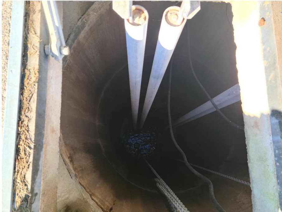
LS #5: Locks Road - Inside of Wet-Well
