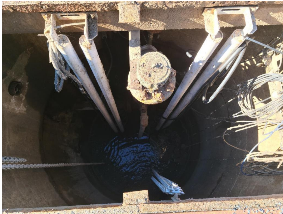
LS #3: Horne Settlement – Inside of Wet-well
