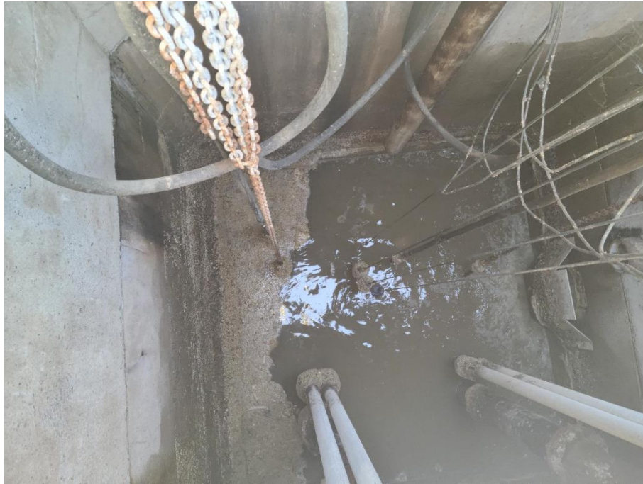
LS #7: Curley Portables - Inside of Wet-Well
