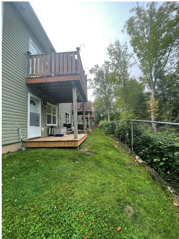
Rear Yard of Two Storey Buildings
