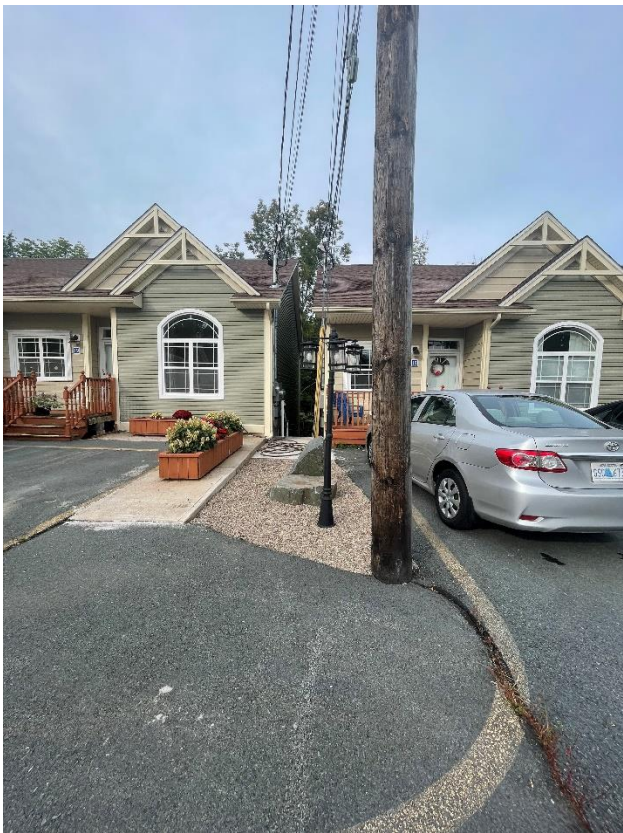
Stairwell Between Buildings
