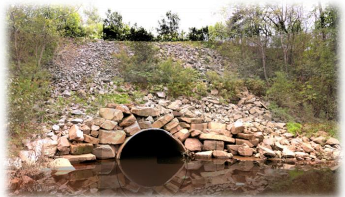
Figure 1 Inlet to CN Railbed Culvert (Oct 2023)
