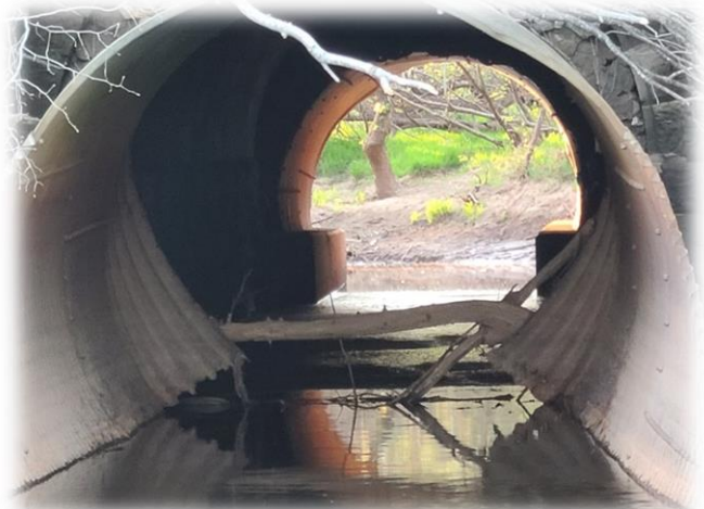
Figure 2 Outlet to CN Railbed Culvert (May 2024)
