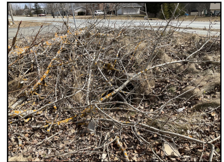
Photo 6: Tree blocking inlet
