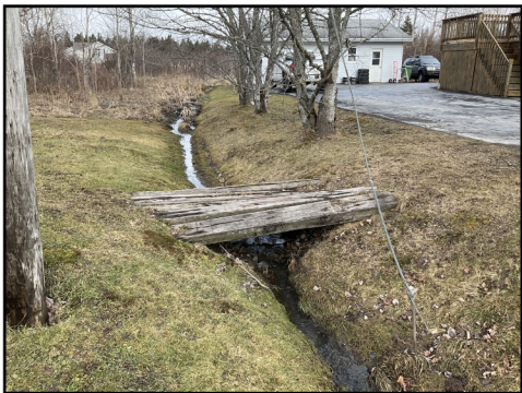
Photo 3: Grassy swale flowing into culvert
