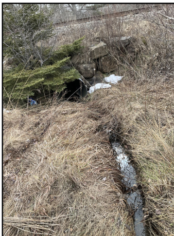
Photo 2: Downstream channel flowing to CN Culvert 13
