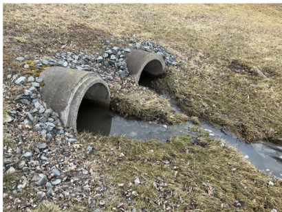
Photo 4: Twin concrete culvert outlets
