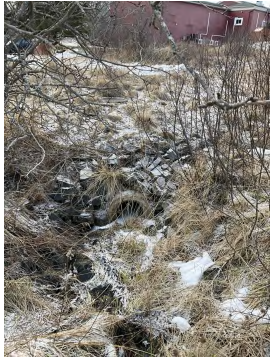
Photo 1: Culvert flowing from Enfield Manor
