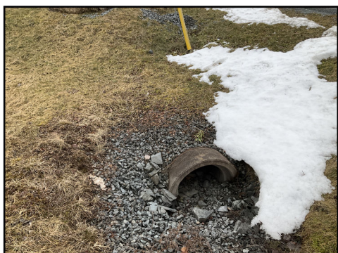
Photo 3: Inlet of 450mm concrete culvert
