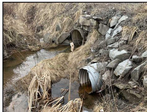
Photo 2: Outlet of concrete and steel culverts
