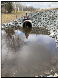
Photo 1: Outlet of culvert
