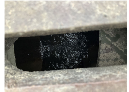
Photo 6: Catch Basin connected to culvert
