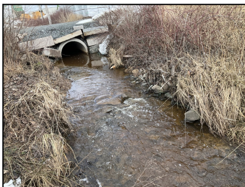
Photo 2: Upstream flow to culvert
