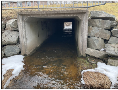
Photo 1: Inlet to culvert
