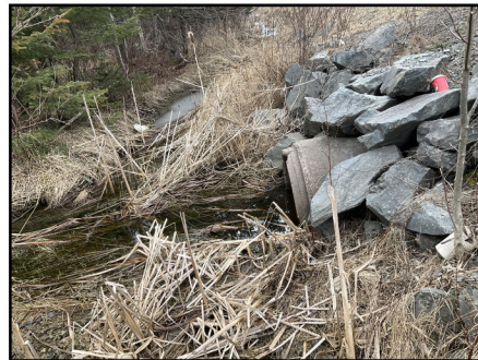
Photo 5: Outlet of culvert
