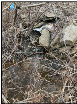
Photo 1: Outlet of culvert
