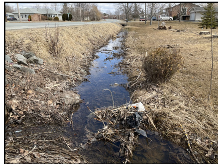
Photo 5: Downstream channel of Culvert 69A
