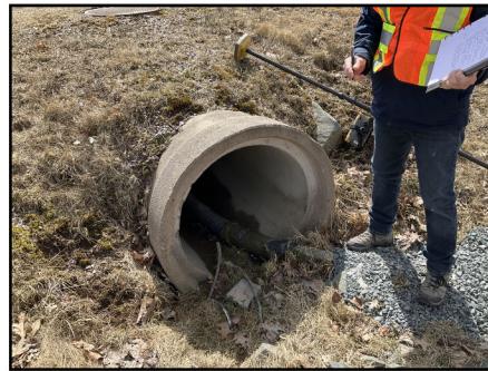
Photo 2: Inlet to culvert with perforated pipe
