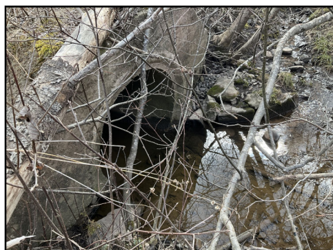
Photo 2: Inlet to culvert
