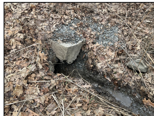
Photo 3: Outlet of culvert
