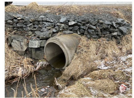
Photo 3: Outlet of pipe with restored head-wall
