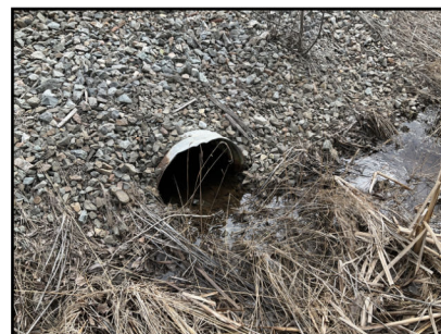
Photo 4: Inlet to culvert
