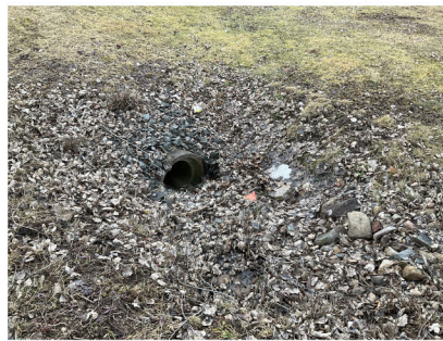
Photo 2: 400mm culvert on west side of upstream manhole
