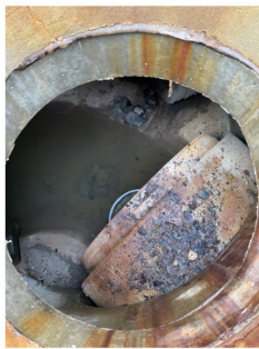
Photo 1: Inside of Catch Basin Manhole connected to culvert
