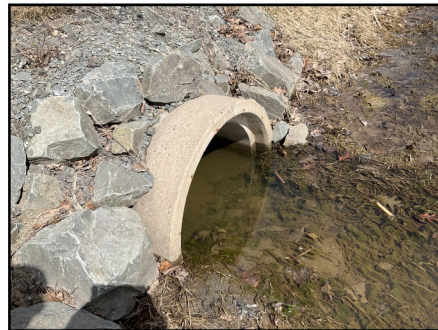
Photo 5: Outlet of culvert
