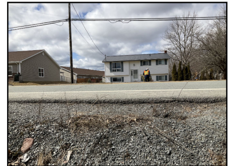
Photo 3: Seniors complex upstream drainage area
