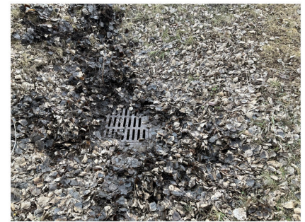
Photo 3: Catch basin on west side of culverts
