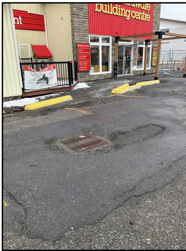
Photo 1: Catch Basin connected to culvert located in Home Hardware Parking Lot
