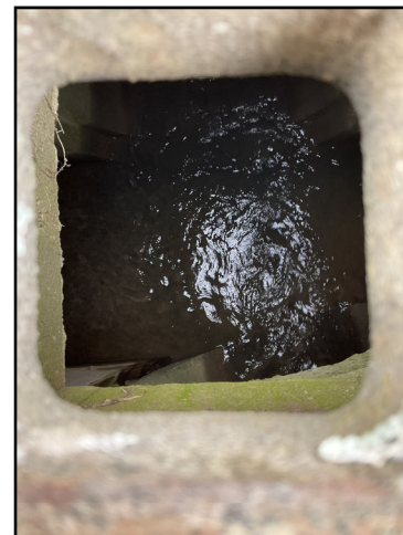
Photo 3: Inside of upstream catch basin showing flow into pipe
