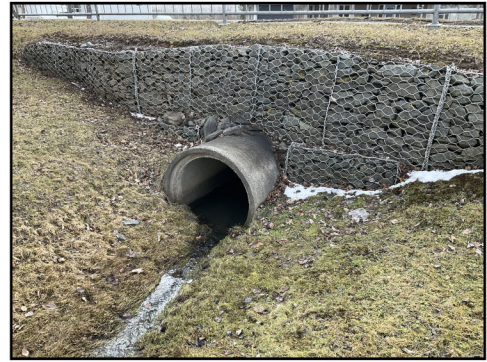
Photo 2: Inlet to culvert
