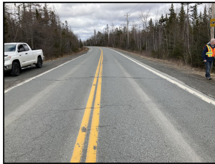
Photo 2: Road cross-section above culvert looking Northeast
