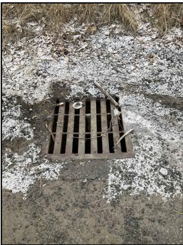
Photo 1: Catch basin on East side of Highway 2.
