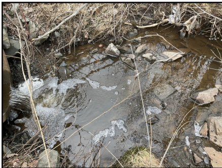
Photo 1: Outlet area of culvert
