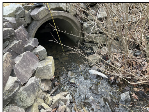
Photo 4: Inlet of culvert
