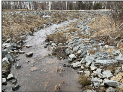
Photo 3: Realigned upstream tributary
