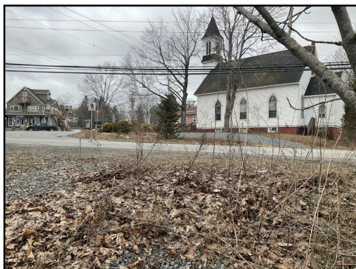
Photo 2: Looking at roadway from outlet of culvert
