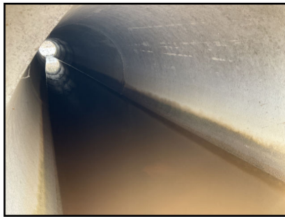
Photo 1: Inside of culvert looking upstream
