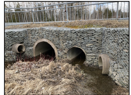
Photo 3: Inlet to culverts with new gabion basket
