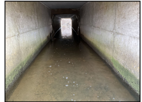
Photo 6: Inside of culvert looking downstream
