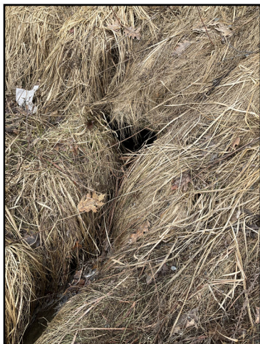
Photo 1: Outlet of culvert
