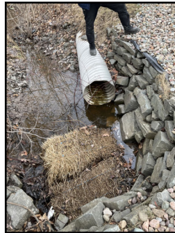
Photo 5: Steel culvert flowing into Culvert 59
