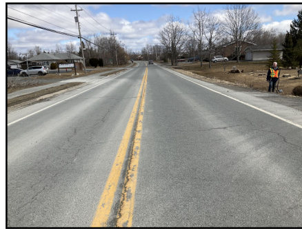
Photo 2: Road cross-section above culvert
