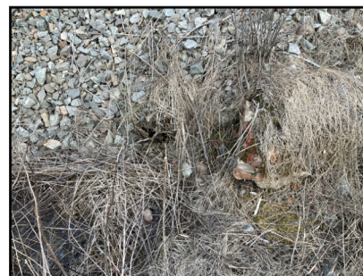
Photo 4: Inlet to culvert
