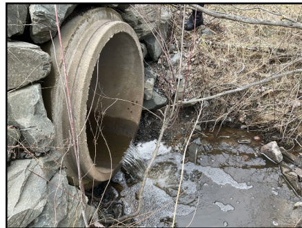
Photo 2: Outlet of culvert with rock head-wall
