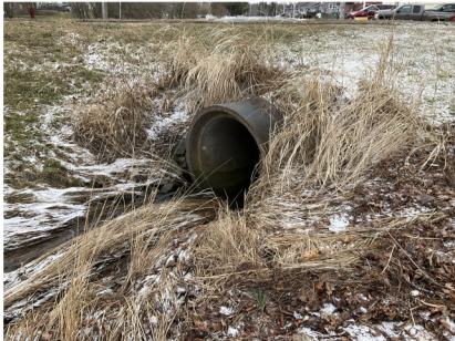
Photo 4: Inlet of culvert
