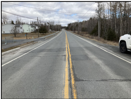
Photo 1: Road cross-section above culvert (looking Northeast)
