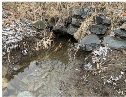
Photo 2: Outlet of culvert
