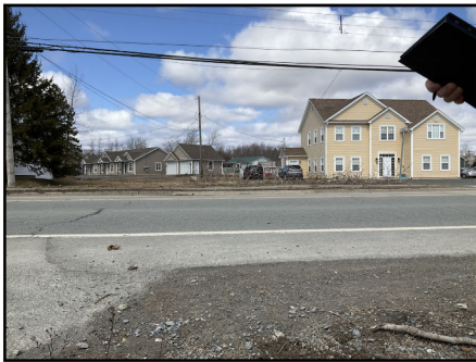
Photo 1: View of area which flows through culvert
