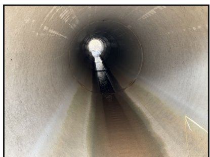
Photo 1: Inside of culvert looking upstream
