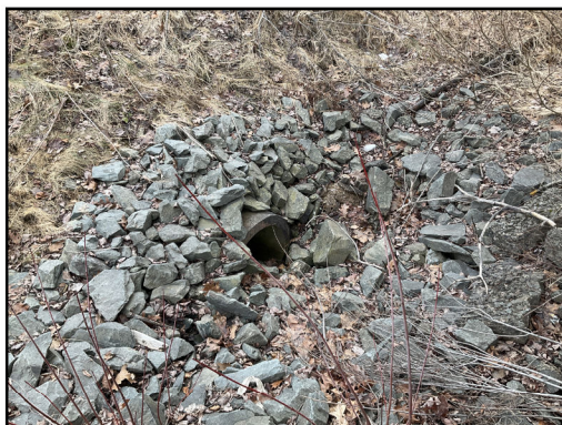
Photo 2: Inlet of culvert
