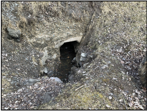
Photo 1: Outlet of culvert to 450mm pipe to the southeast
