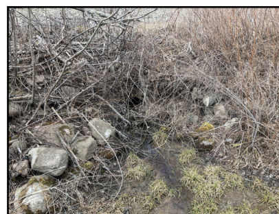
Photo 2: Downstream drainage area looking at outlet of culvert
