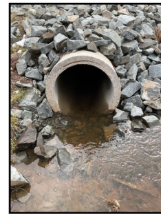
Photo 2: Inlet of culvert
