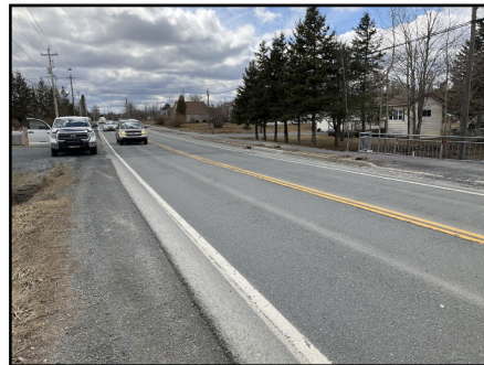
Photo 2: Road cross-section above culvert (looking Southwest)
