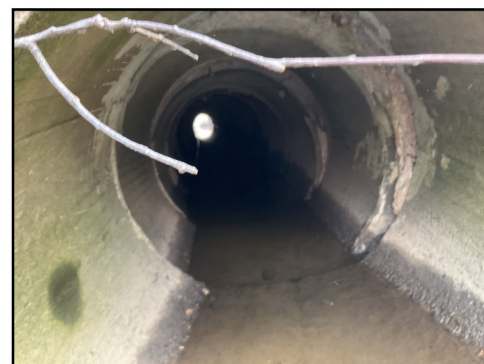
Photo 3: Inside of culvert looking downstream
