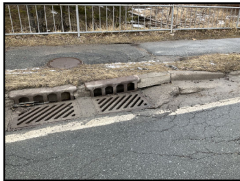
Photo 5: Storm sewer connected to culvert
