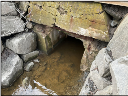
Photo 4: Downstream headwall
