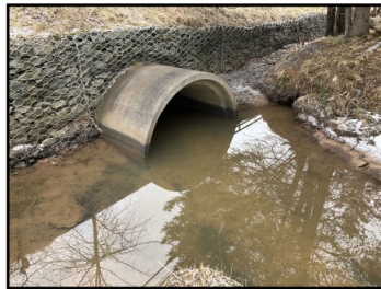
Photo 6: 1500mm concrete inlet
