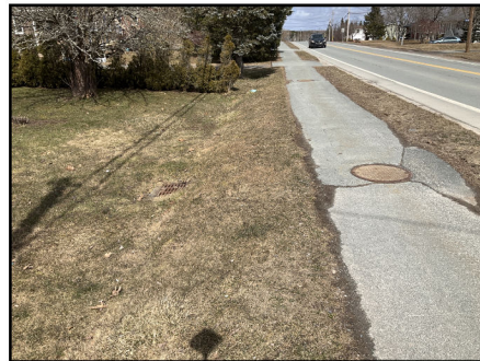
Photo 5: Catch basin in local yard upstream
