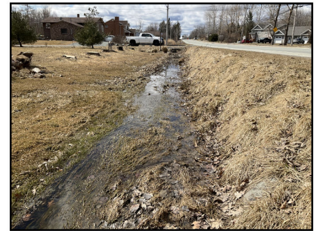
Photo 3: Downstream channel looking towards Culvert 69
