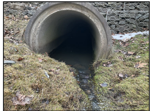
Photo 4: Inside of culvert looking downstream
