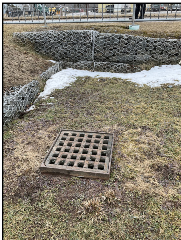
Photo 1: Upstream catch basin
