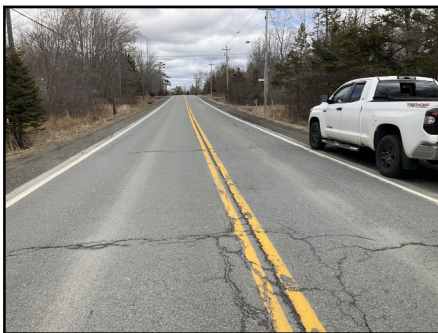
Photo 1: Cross-section of road above culvert looking Northeast
