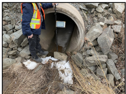
Photo 3: Inlet of culvert
