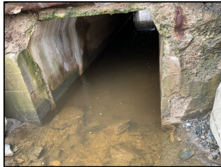
Photo 5: Outlet of culvert
