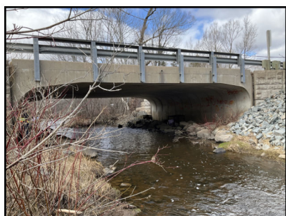
Photo 1: Conspan from downstream side
