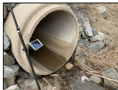
Photo 2: Outlet of culvert
