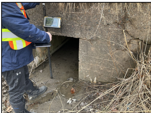
Photo 1: Outlet of culvert
