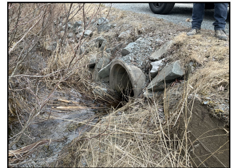
Photo 6: Inlet to culvert
