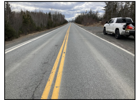
Photo 3: Road cross-section of culvert looking Southwest
