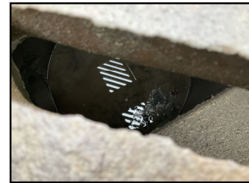
Photo 8: Inside of catch basin connected to culvert
