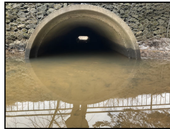
Photo 7: Inside of the culvert looking downstream
