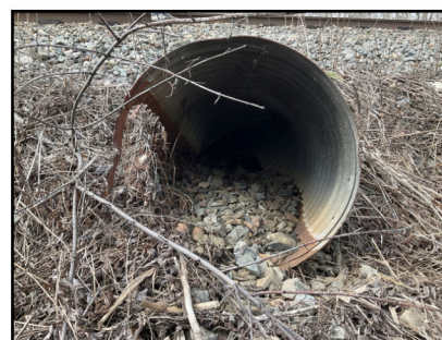
Photo 2: Outlet of culvert
