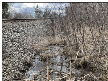
Photo 3: Area upstream of culvert along railway
