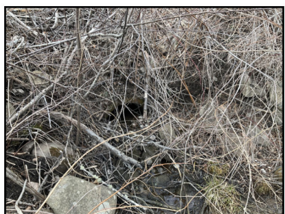
Photo 1: Outlet of culvert
