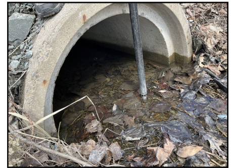
Photo 3: Outlet of culvert
