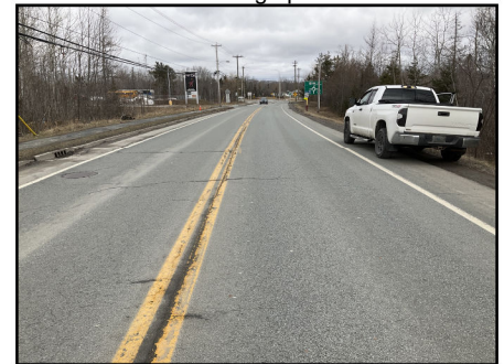
Photo 6: Road cross-section above culvert
