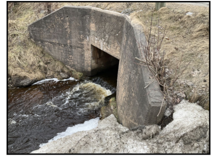
Photo 2: Outlet of culvert
