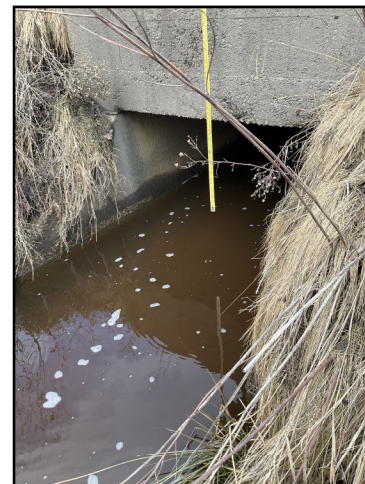
Photo 3: Outlet of culvert
