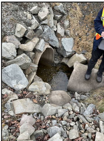
Photo 2: Outlet of pipe to pipe flowing under Truck Yard
