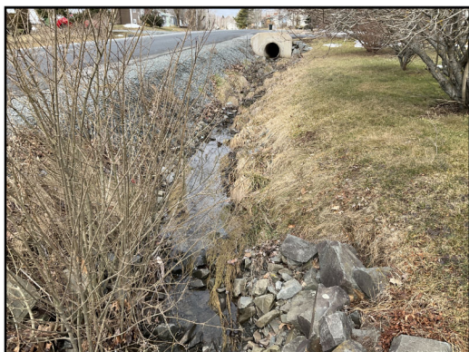
Photo 3: Drainage ditch on side road flowing to culvert
