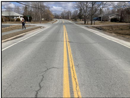
Photo 4: Road cross-section above culvert
