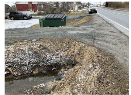
Photo 3: Ditching around outlet of culvert
