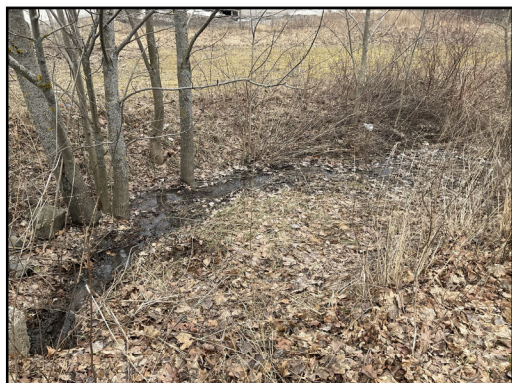
Photo 1: Flow from culvert after clearing debris
