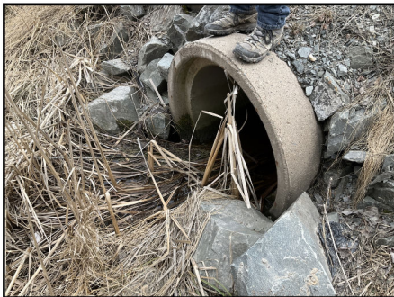
Photo 4: Inlet to culvert
