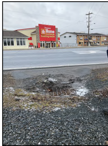
Photo 2: Catch Basin connected to culvert located across the road from Home Hardware
