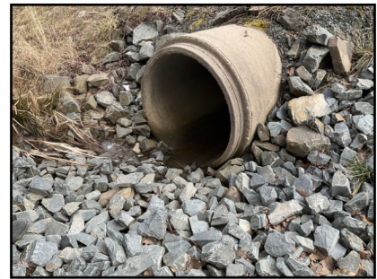
Photo 2: Inlet of culvert with rip-rap channel
