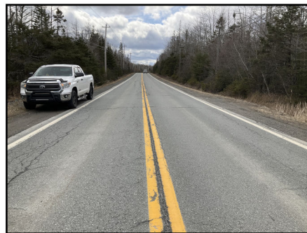
Photo 2: Cross-section of road above culvert looking Southwest
