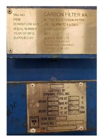
Figure 2.3 – GAC Filter Name Plate
