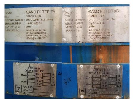
Figure 2.1 – Sand Filter Name Plates
