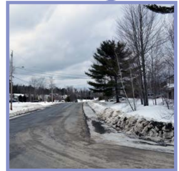
Older roads within subdivisions have no sidewalks. At some locations culverts, soft shoulders and snow buildup may force AT into roadway.
