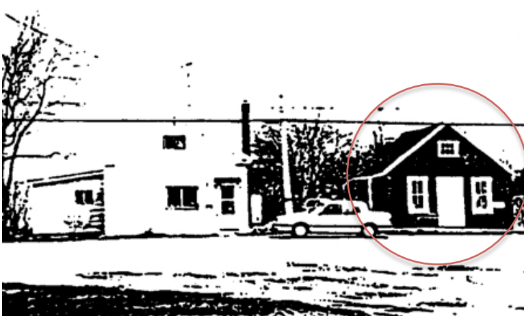
[Figure 4] Demolished Building 1
